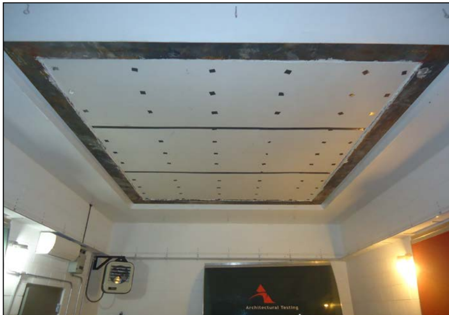
Receive Room View of Test Specimen Installation
