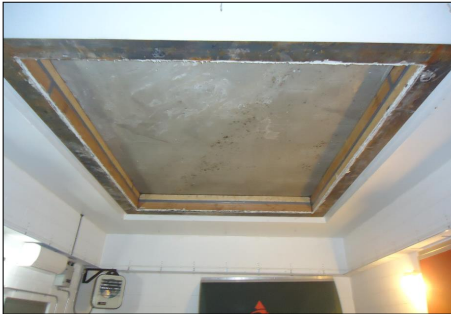
Receive Room View of Test Specimen Installation
