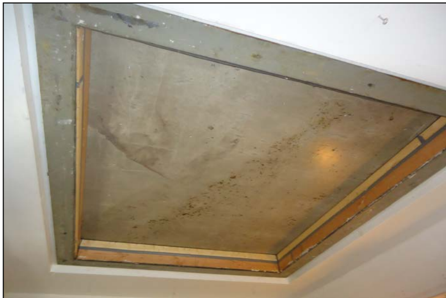
Receive Room View of Test Specimen Installation
