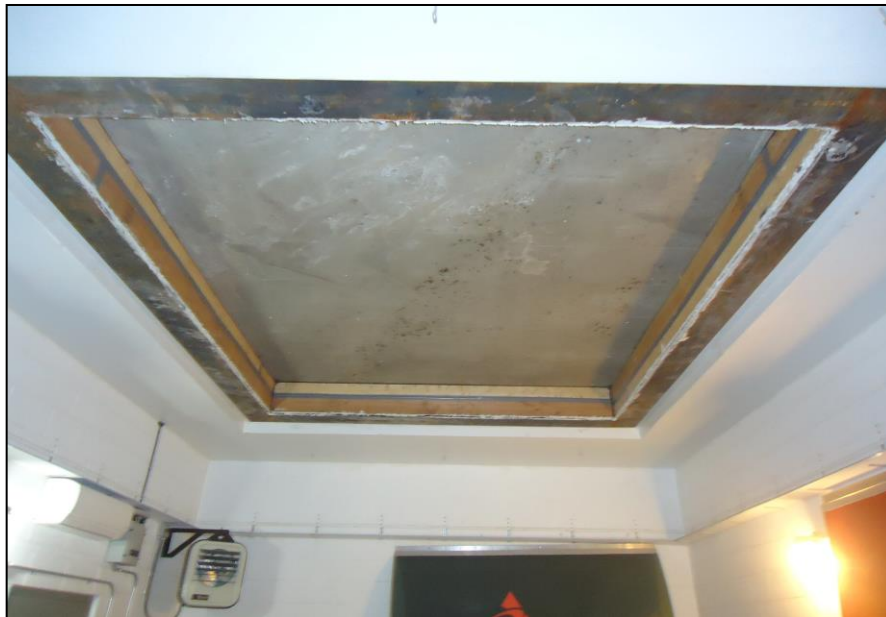
Receive Room View of Test Specimen Installation
