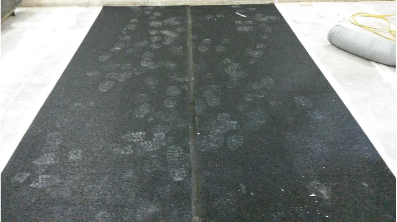
Figure 3 – Detail of underlayment installed on concrete slabs.
