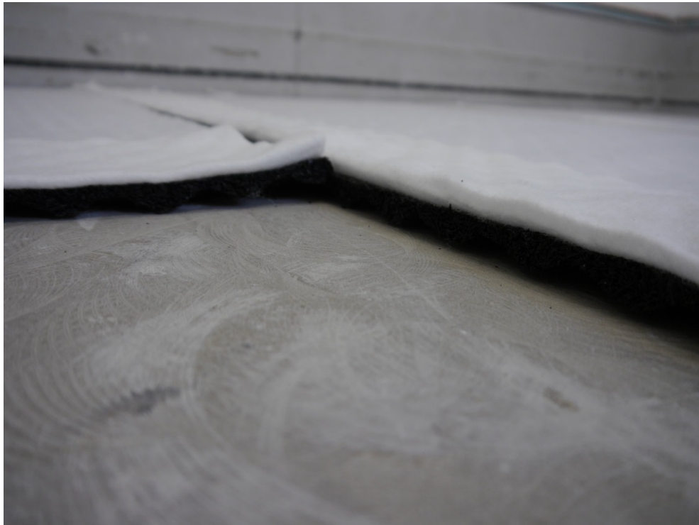
Figure B.1. Laying of the sound insulation layer Regupol® sound and drain 22 on the uncovered concrete floor.
