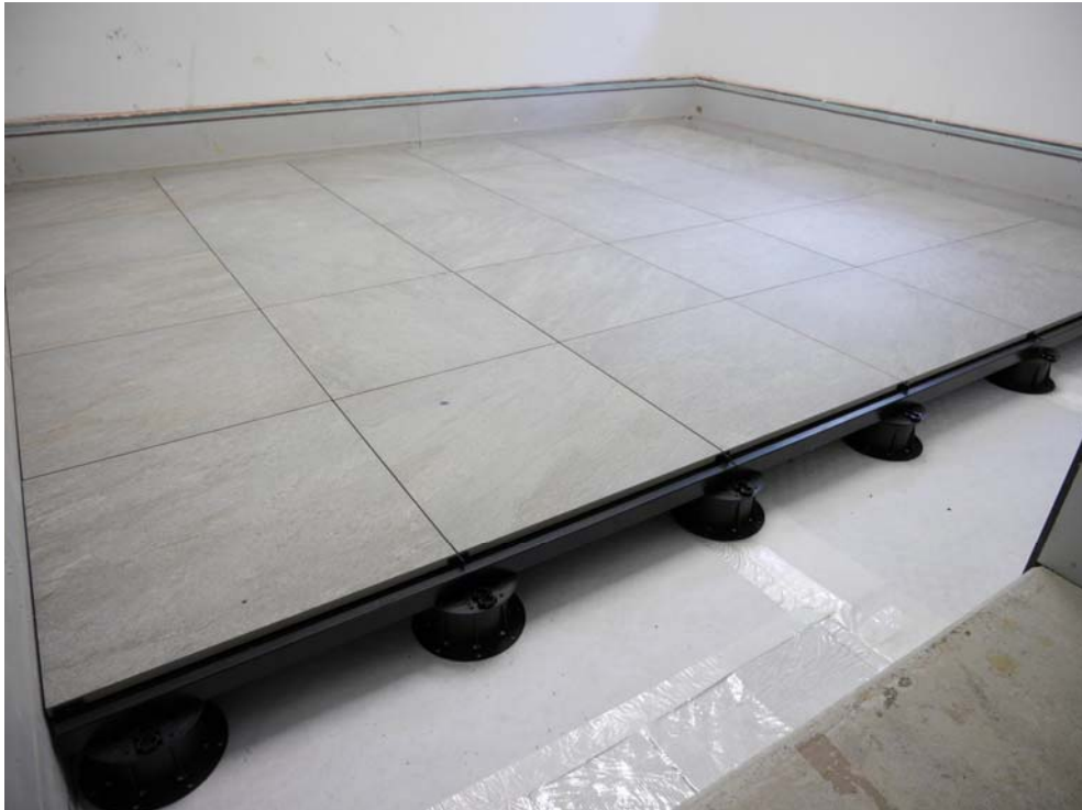
Figure B.5. Test setup in the ceiling test facility: ready for testing.
