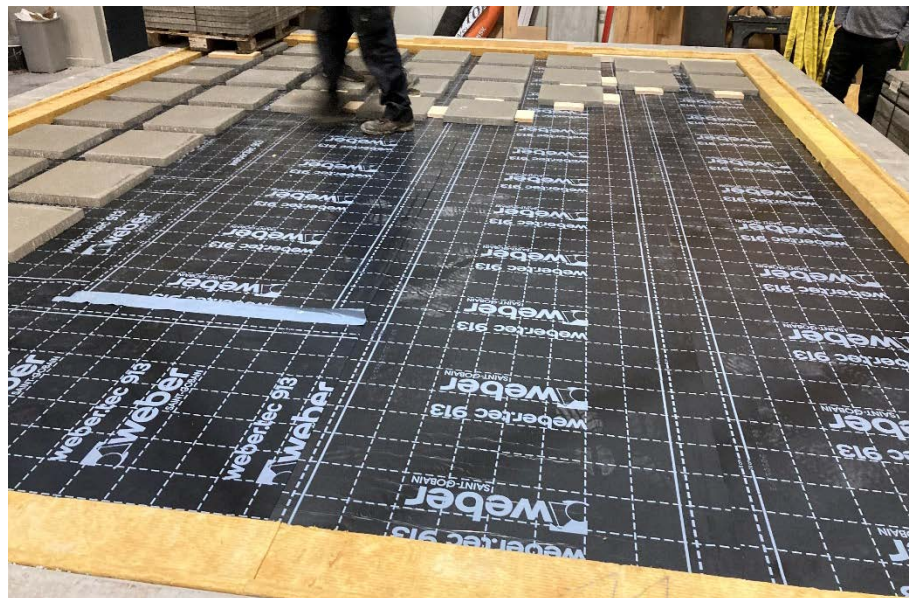
Fig. 2: Laying the concrete tiles (400 × 400) mm 2 on the cold self-adhesive membrane.
