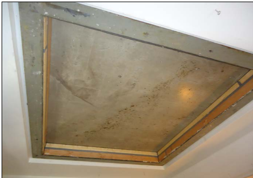
Receive Room View of Test Specimen Installation
