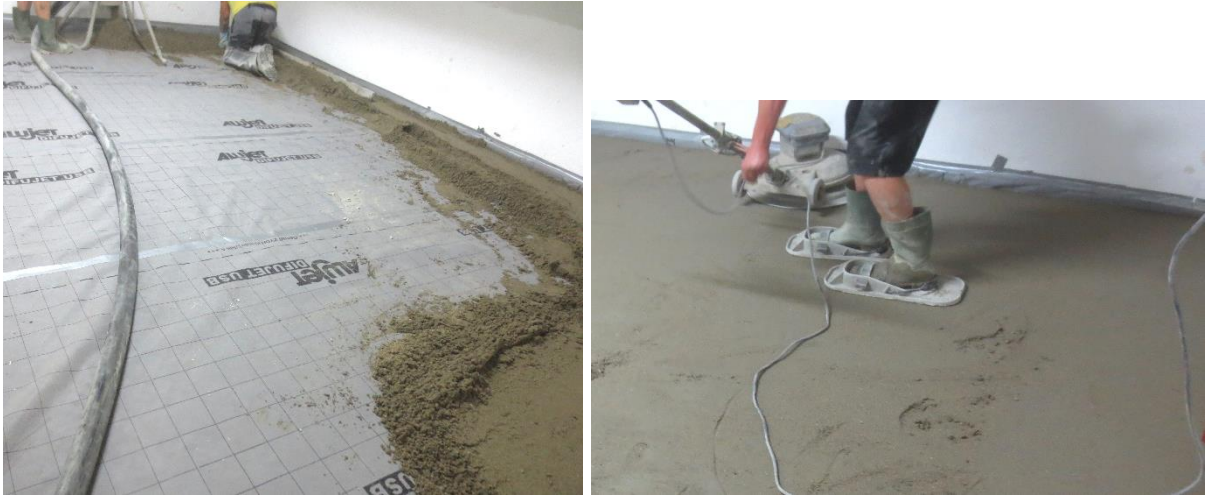
Figure A 2.4: situation during mounting - cement screed
