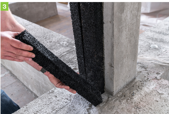
Loosely attach the outer strip REGUPOL INODIS vertical .
