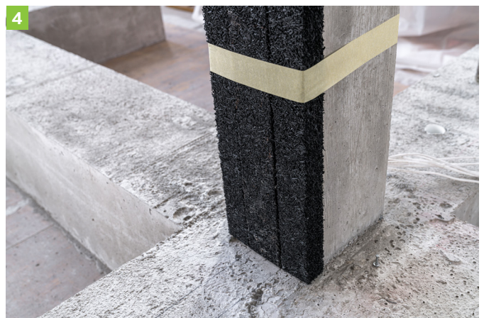
Fix the REGUPOL INODIS vertical with a tape.
