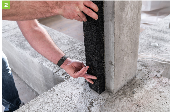
Glue the middle strip REGUPOL INODIS vertical .
